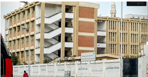
Figure (6). Sun breakers on the western and southern facade. (Author., 2023)
